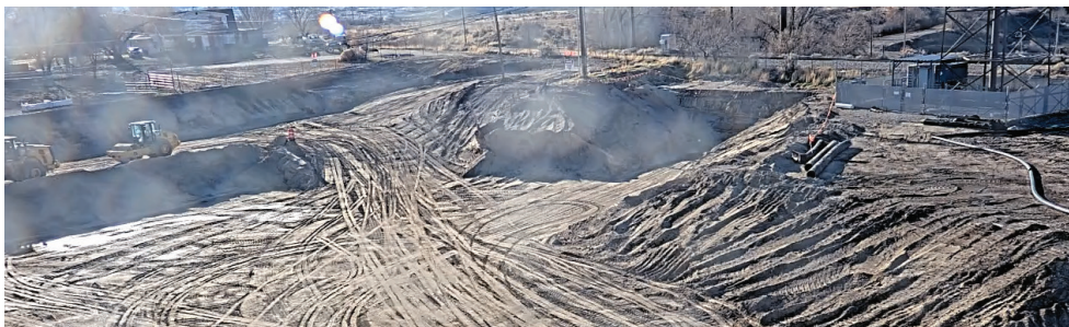
Image of construction property looking west.
