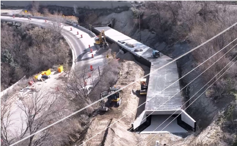
New culvert installed on 14600 South. Photo credit: Kevin Thompson
