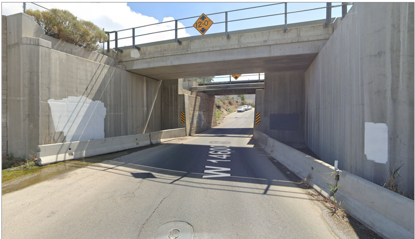
Figure 1. Existing Railroad Bridge and 14600 South Underpass
